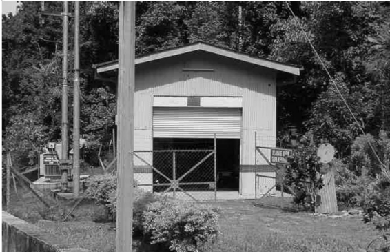
Figure 3: Pelton Type Turbine and Power House
