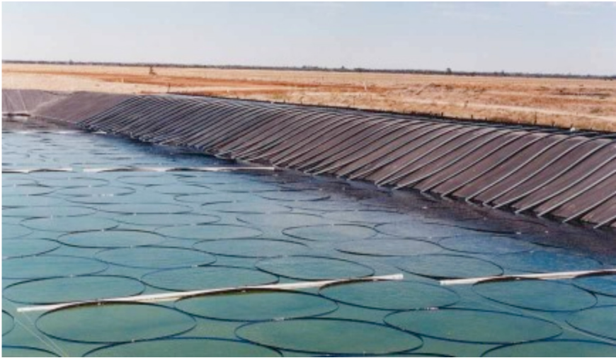
Figure 4. Solar pond at Kerang (Northern Victoria, Australia) showing the plastic rings used for wind control and pipes crossing the pond -used as heat exchanger.
