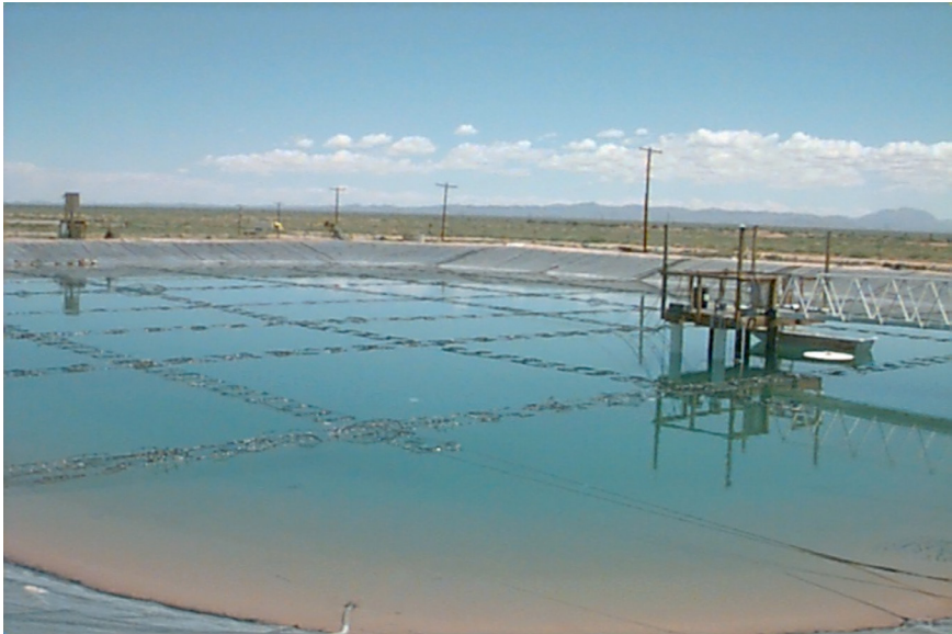
Figure 14. Dead Sea Solar Pond
