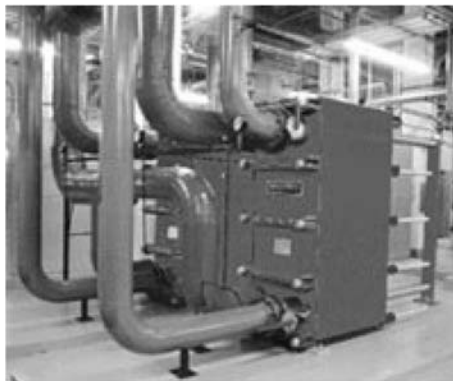
Figure 1. Plate & Frame Piping
