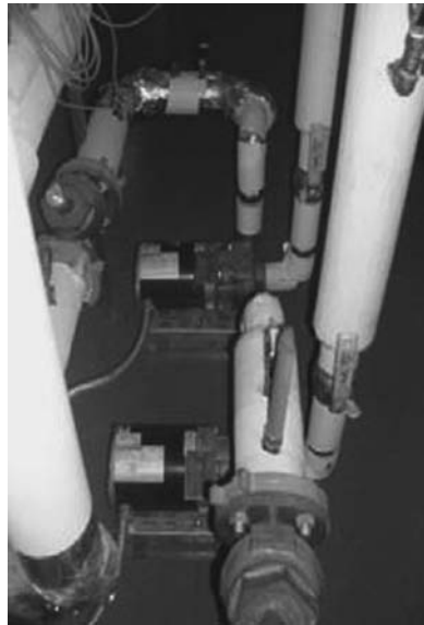
Figure 4. Circulating Pumps
