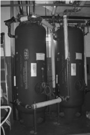
Figure 3. DHW Tanks
