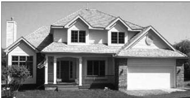
Figure 16. Wood Gasifier Demonstration Home in Madison, Wisconsin
