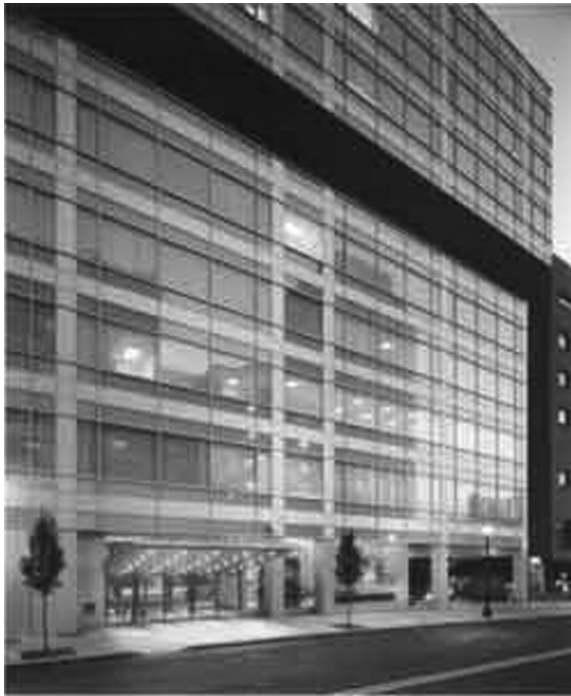
Figure 5. At Montefiore Medical Center in the Bronx NY, 90% of the Patient Areas are Powered by CHP.
