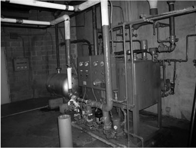
Figure 4. Thermal Heat Sink Tie-in at a Health Care Facility for Use with CHP.
