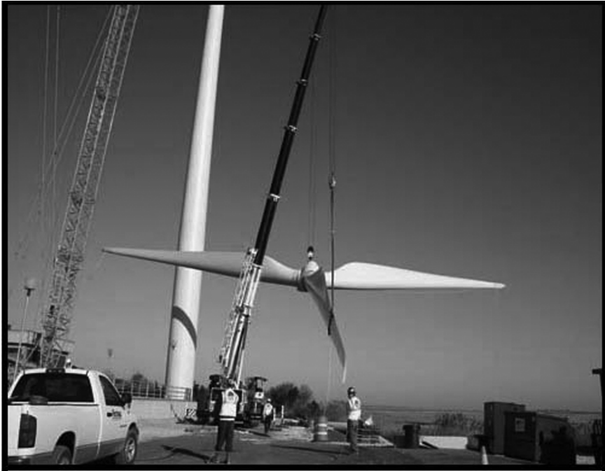
Figure 3. Wind Turbine Construction Photo
