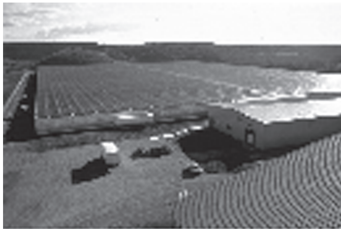
Figure 17. Example of a Large CHP Plant
