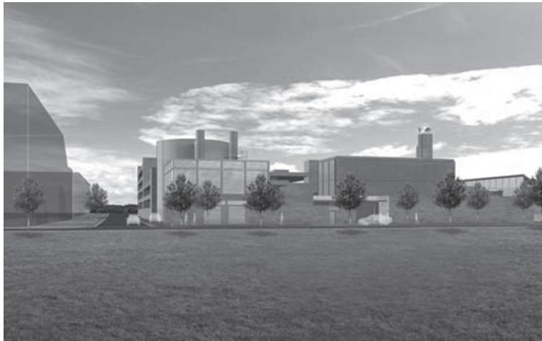
Figure 1. Rendering of the Dell Children's Medical Center of Central Texas. Rendering Courtesy of Karlsberger
