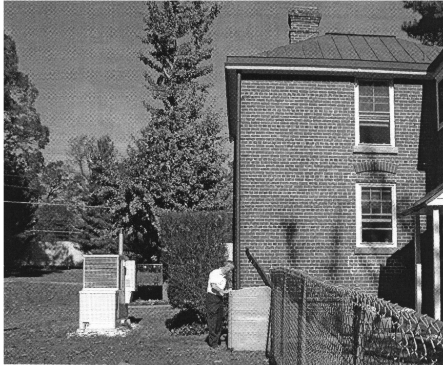
Figure 3. Demonstration PEM Fuel Cell-based CHP unit (left) at Fort McPherson.
