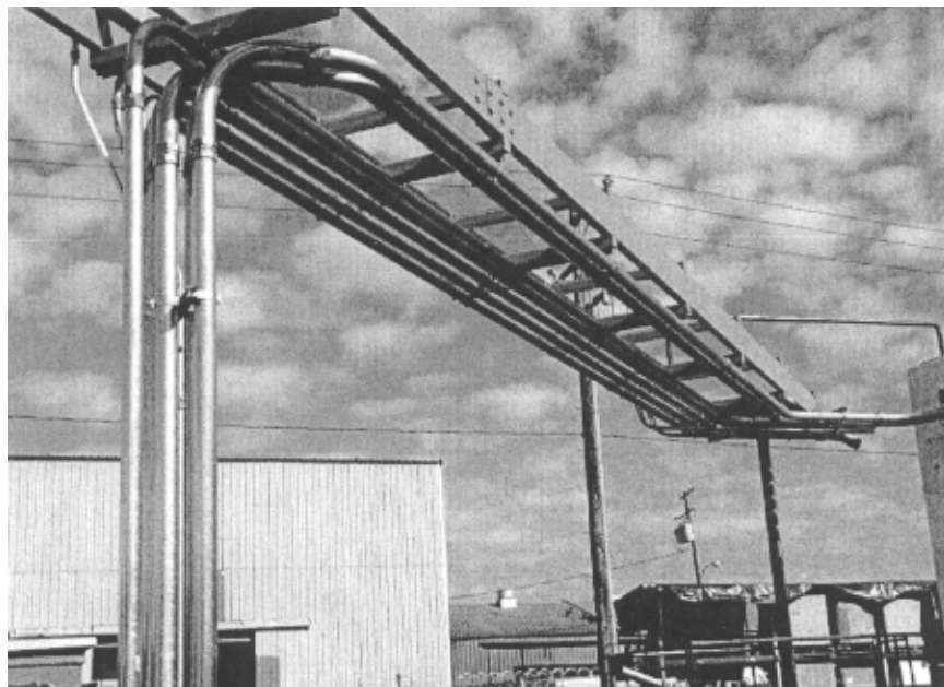
Figure 10. Service trestle Medway Plastics
