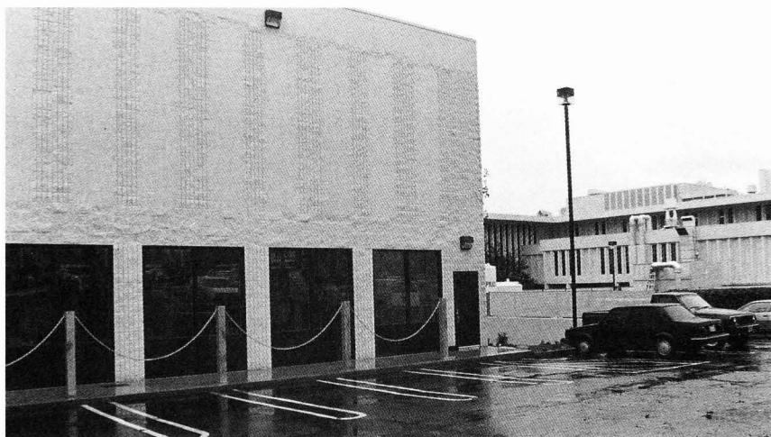
Figure 5. From the parking lot, the four engine/generator trains can be seen through large plate glass windows. If the engines ever have to be removed, the windows and their frames will be removed.
