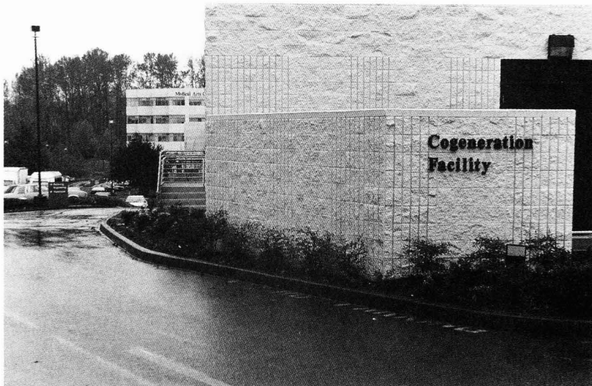
Figure 4. The cogeneration facility at the Valley Medical Center is housed in an attractive building which fits in with the overall architecture of the medical complex.
