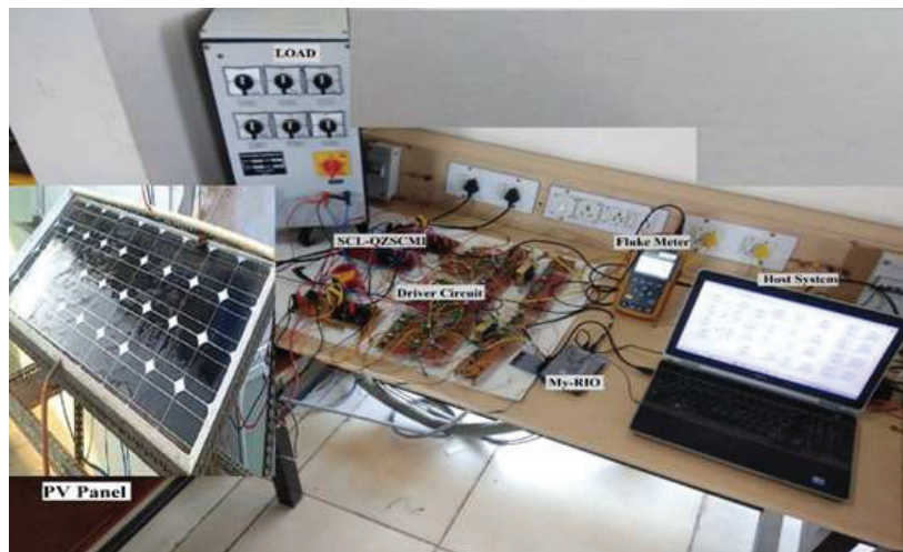
Figure 19 Photograph of the experimental test bench of the SCL qZS-CMI with the PV system.
