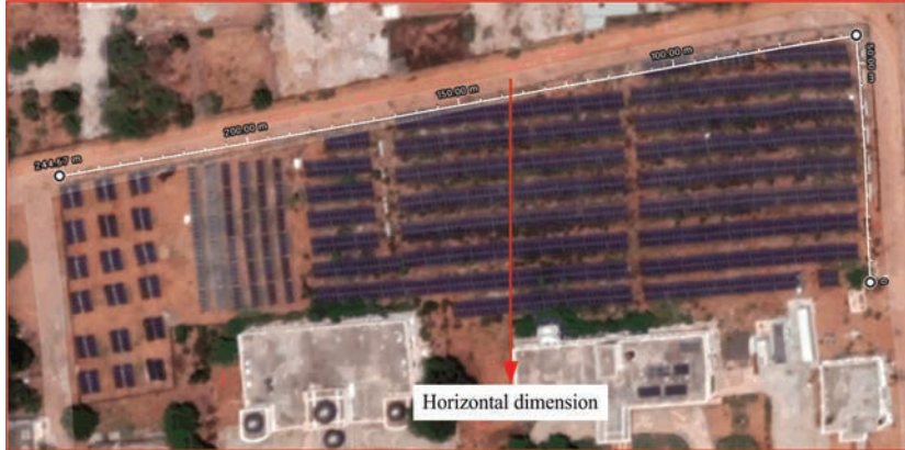
Figure 4 An aerial view of the 500 kW P plant profile.
