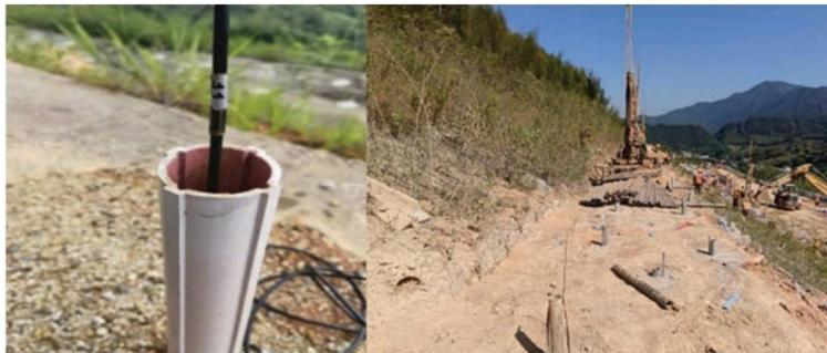
**Figure 10** K738+915~K739+156 section III platform perspective and inclinometer pipe layout.
