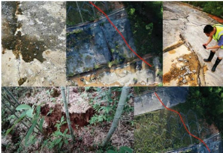
**Figure 4** Cracking of on-site slope and platform.
