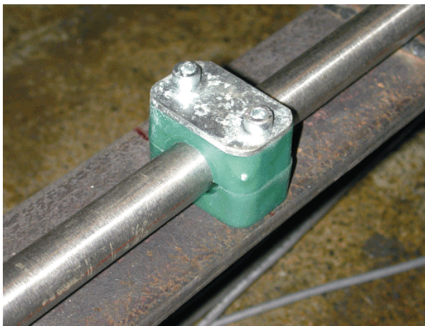
Fig. 2: The bracing of the pipe
