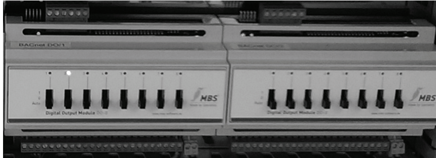
Figure 2 Unused BACnet digital output devices.
