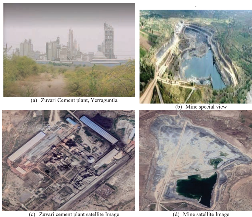
Figure 5 Zuvari cement plant, mine spacial view, plant and mine satellite images.
