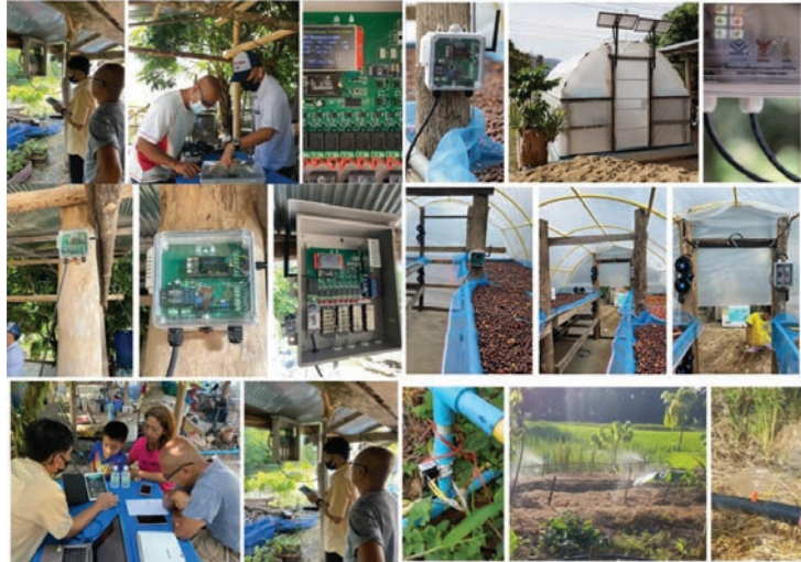
Figure 12 System installation at Cocoa farm, Thailand.
