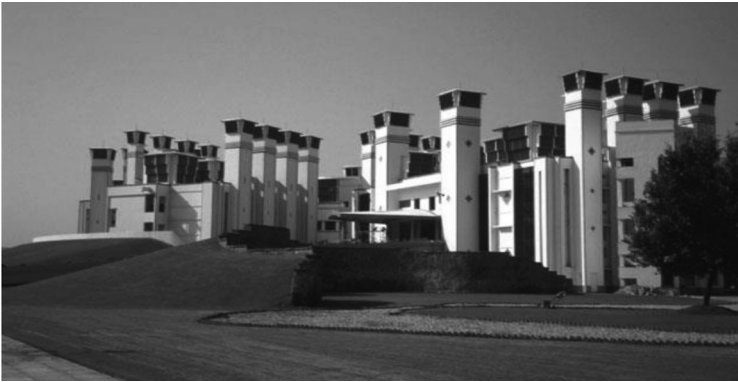
Figure 12. Torrent Research Centre passive down draft evaporative cooling, Ahmedabad (photo courtesy: Abhikram) [52].
