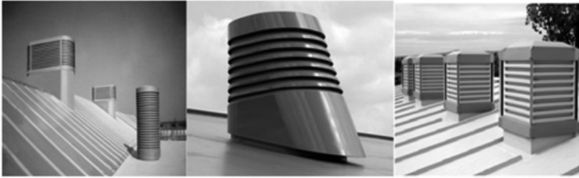
Figure 8. Examples of mono-draft wind catchers [39].
