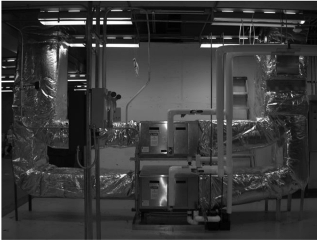
Figure 1. HHS heat pump heat recovery system.
