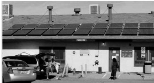
Figure 3. 20 panels of 100 on the Thrift Shop 30 KW Photovoltaic System (1996).
