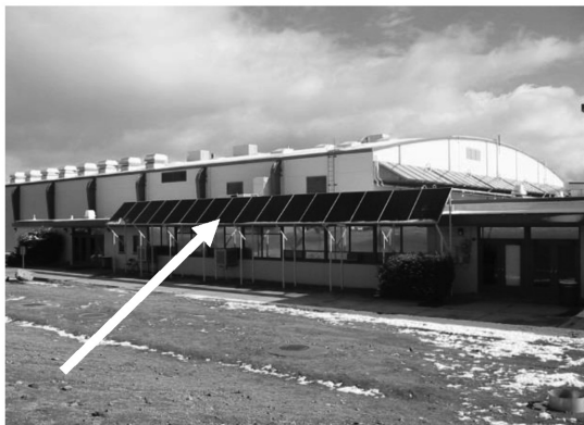
Figure 4. Grid connected photovoltaic system (4.8 kW at Barnes Field House) 1998.
