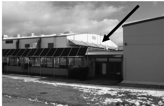
Figure 2. Solar Domestic Hot Water System at Barnes Field House (1981).
