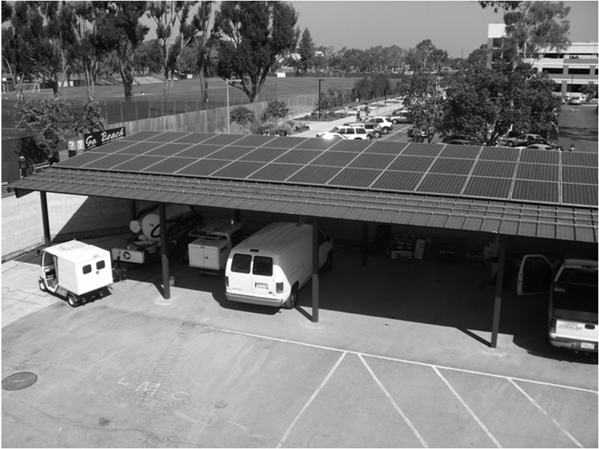
Figure 1. CSU Long Beach solar carport during construction
