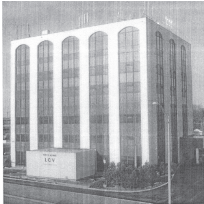
Figure 1. Demonstration Building Following Film Installation
