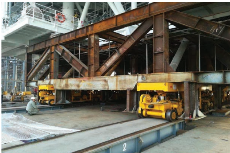
Figure 2 Hydraulic trolley and specialized bracket.
